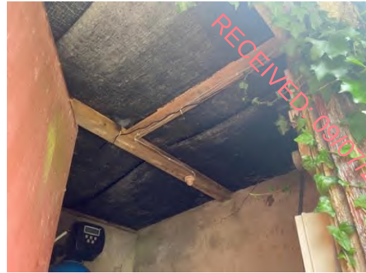
Plate 4-21 Felt underlining within shed.
