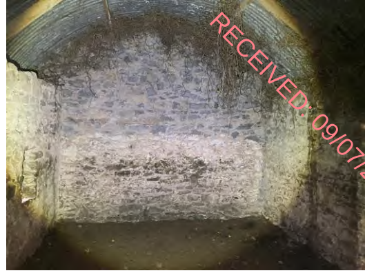
Plate 4-27 Interior of shed.
