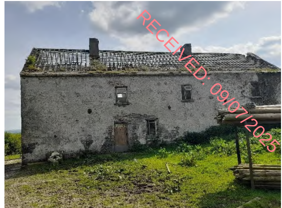
Plate 4-2 North aspect of farmhouse
