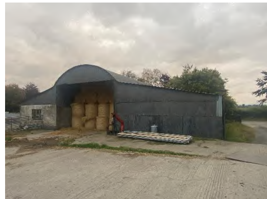
Plate 4-15 Corrugated metal hay storage shed.
